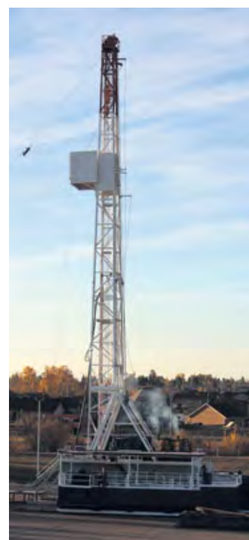
Northern Lights College's simulated well site training facility in Fort St. John, B.C., includes a decommissioned drilling rig. SUPPLIED
